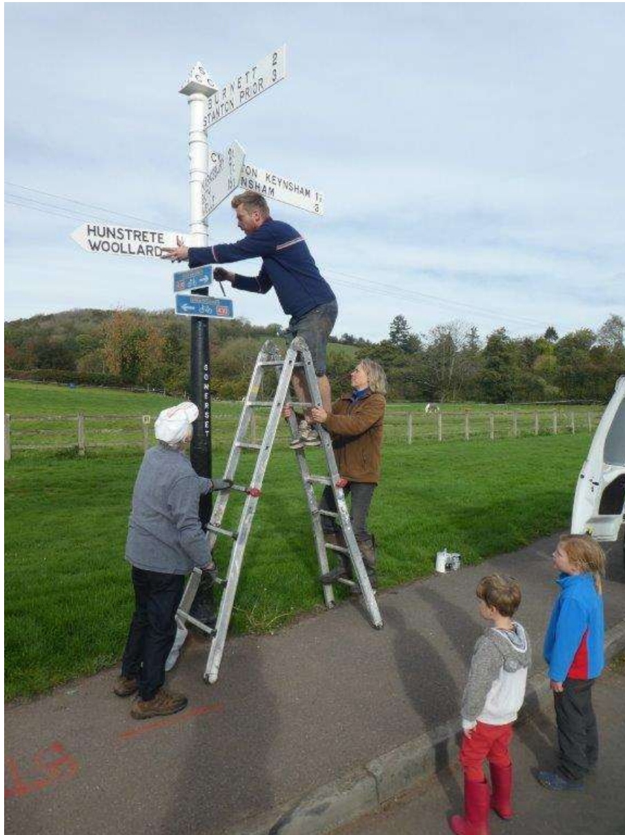
The Restored Millennium Green Fingerpost is put back in position
