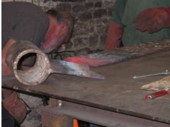
Pieces are now ready for arc welding together
