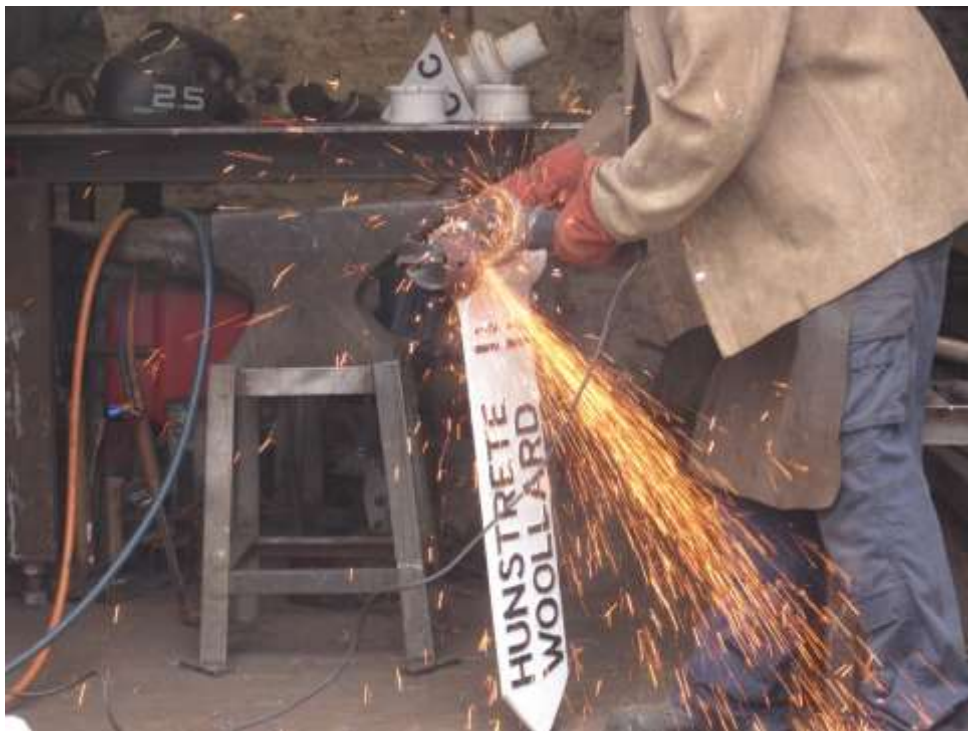
Cutting away the exposed inner post
